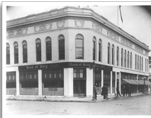
The Modesto Branch in 1917. Image provided by the Bank of America Historical Collection.
