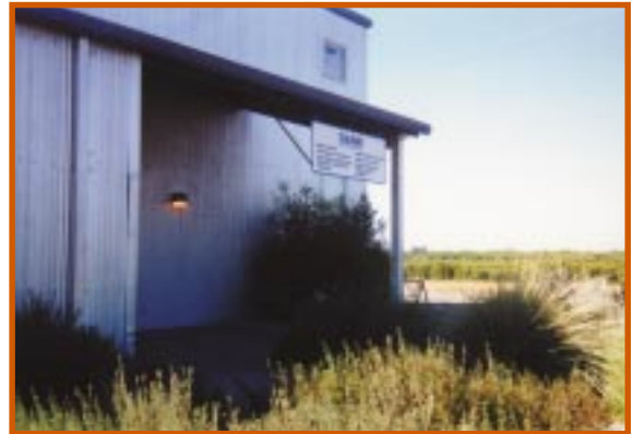
The DANR Building on the UC Davis campus, home to the Small Farm Program.
